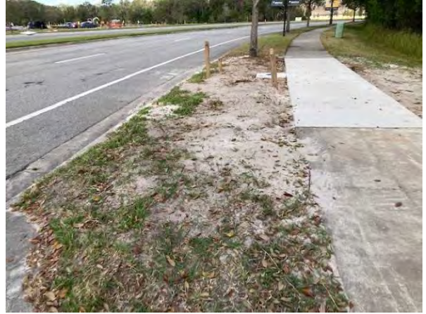
Between side walk and roadway
